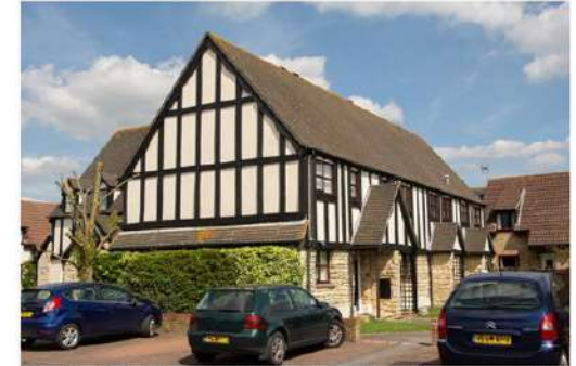
22 to 27 (odd) Field Court, Courtfield Road – 15 th and late 16 th century restored 1985
